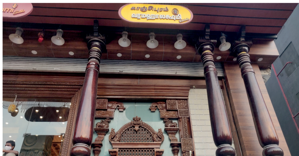
Figure 2: The wooden façade of the Kanchi Vara mahalakshmi Shop
